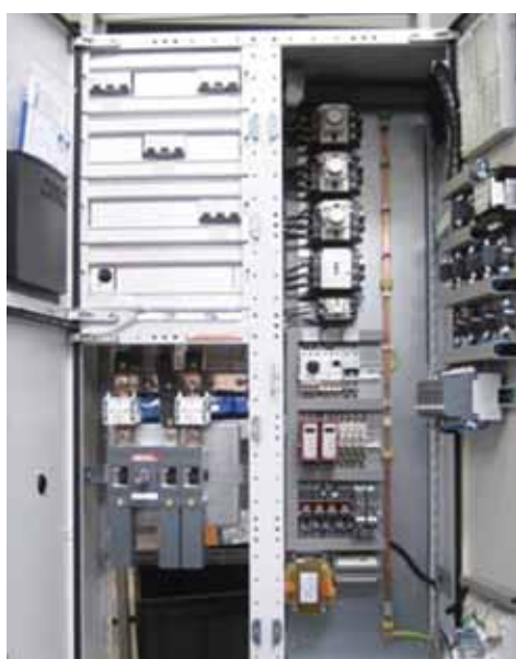
Control panel for the Aalborg EH-S heater
